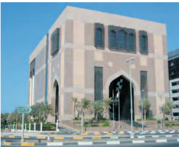
Fund Head Quarters, Abu Dhabi - United Arab Emirates
