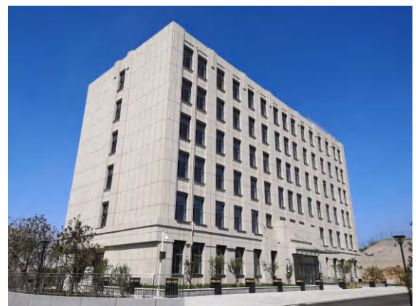
State Grid EHV AC / DC operation inspection center, Qingdao - China
