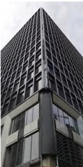
Qiantan Qiyao investment building, Shanghai - China
