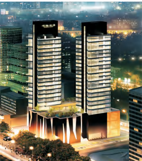
Kunlun Building, Beijing - China
