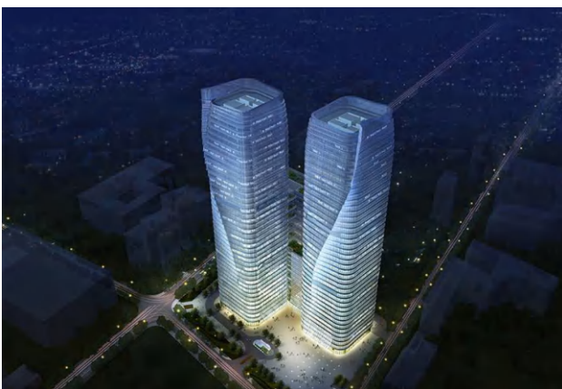
Chuangyi Technology Building, Shenzhen - China
